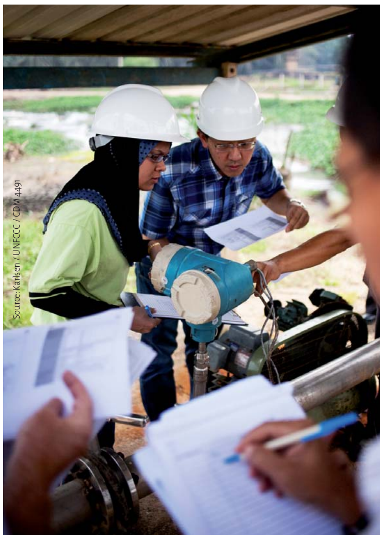
Testing readiness: Wastewater treatment at a palm oil mill in Thailand.
