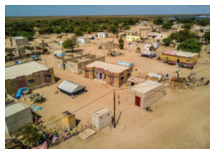
View of ville with the electric installations, region of Saint Louis, Senegal. 31.01.2019.
